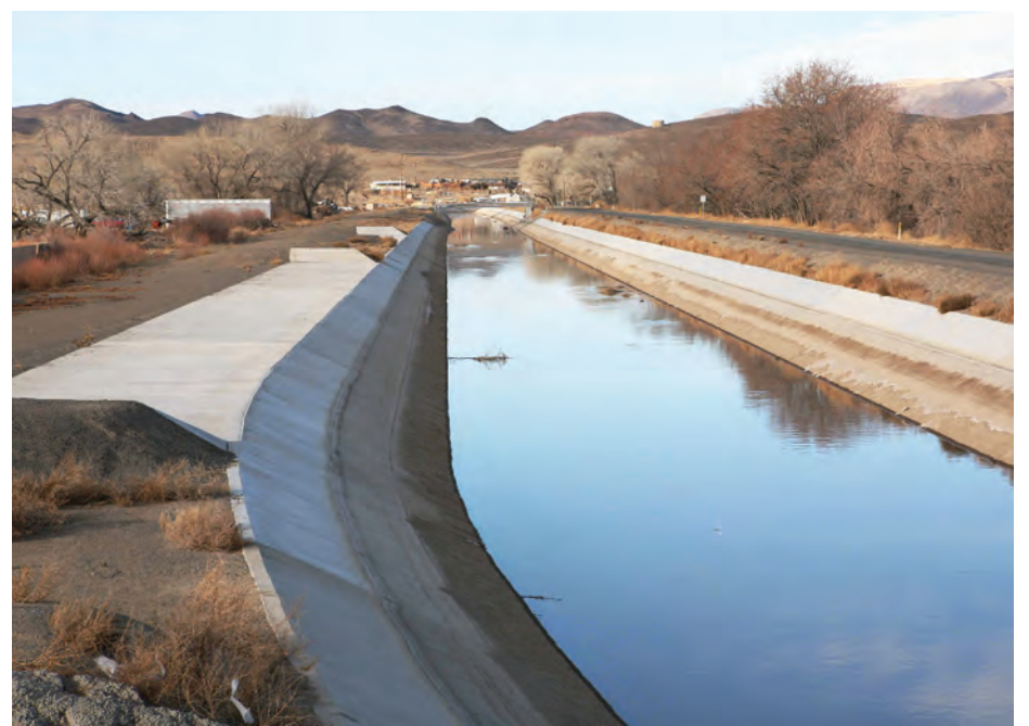
Truckee Canal after lining project.
