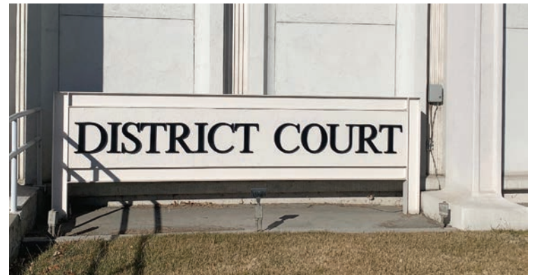
Tenth Judicial District Court Building.
