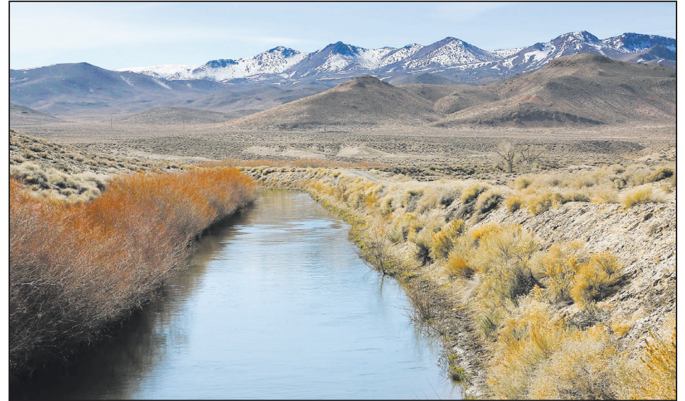
Truckee Canal. Photo courtesy of the City of Fernley.
