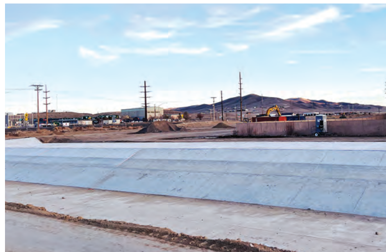
Lined portion of Truckee Canal in Fernley. Photo by Leanna Lehman.
