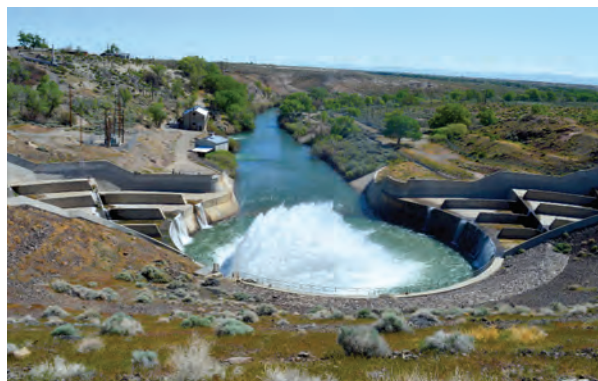
Water being released from Lahontan Dam, generating hydroelectricity. Old and new Lahontan power plants are on the left.
